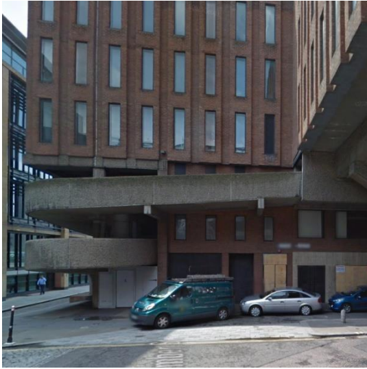
Before (South Side)
